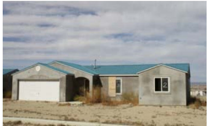
Thousands of single-family homes, abandoned mid-construction, lie vacant in Ship Rock. Photo by Darren Tobia
